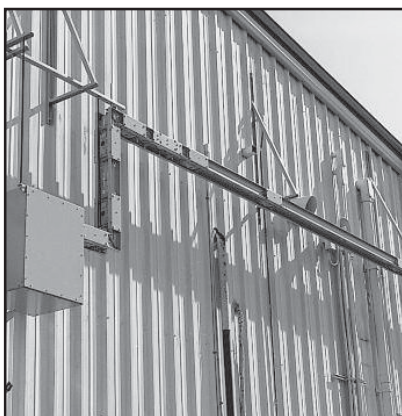
Complete outdoor run of Spectra Series busway.
